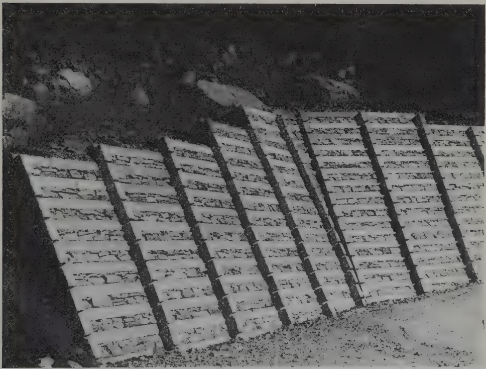
Fig. 8—16. Concrete crib walls, the Tauern Mts., Austria (photograph by Rybář).
