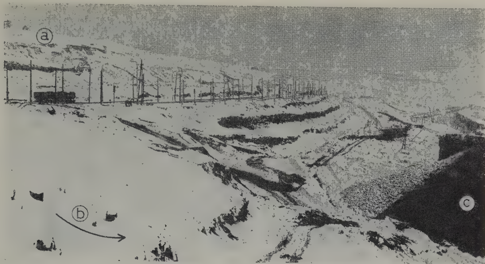
Fig. 13-8. View of slope failure along the slip surface indicated by 8 in Fig. 13-7; a — head scarp, b — direction of movement, c — loading fill.
