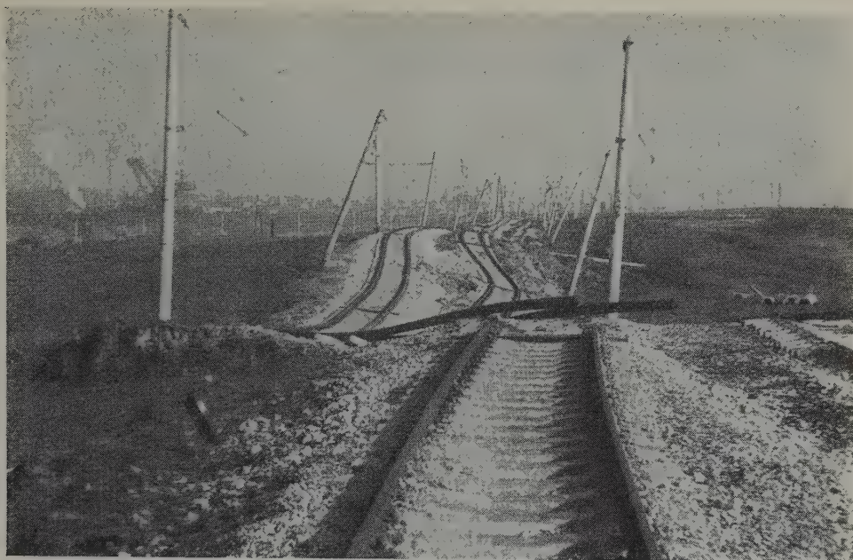
Fig. 1-11. A railway line interrupted by a landslide; Marica-Iztok brown-coal basin in Bulgaria (photograph by Rybář).
