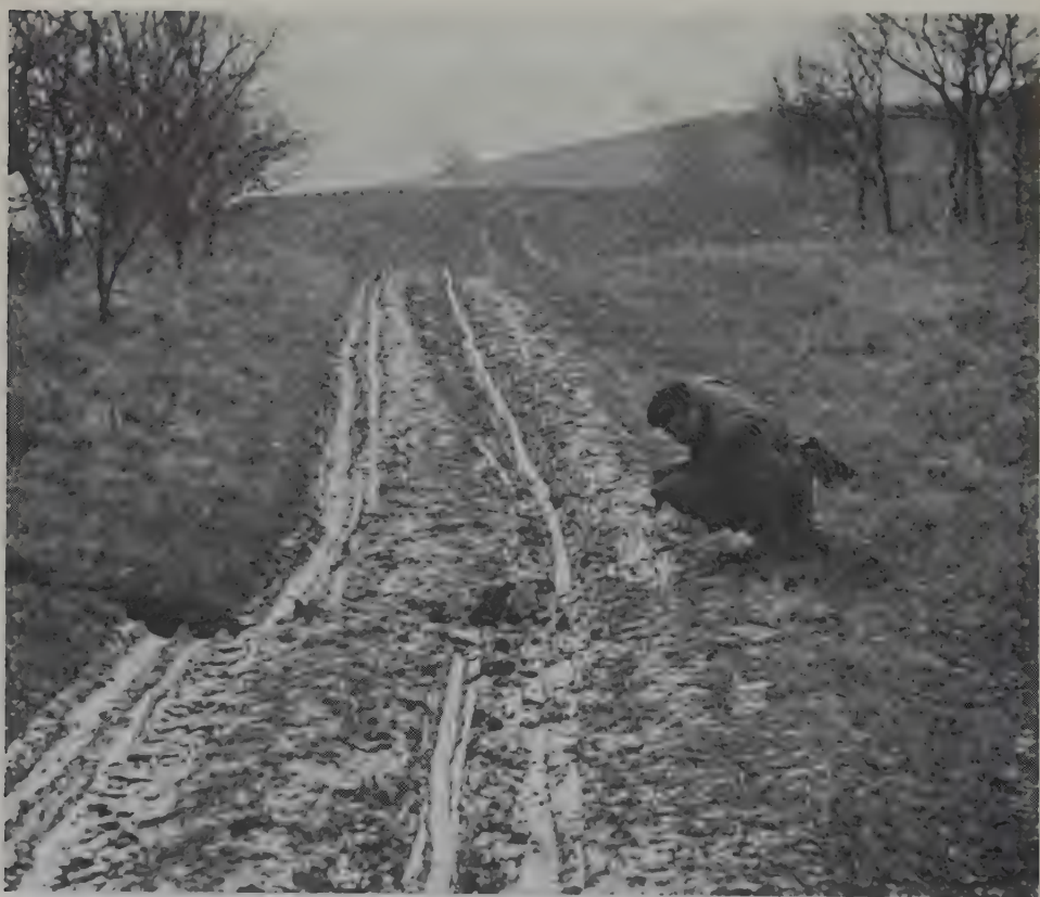
Fig. 3-2. Road dislocated along a crack suggests recent movement (photograph by Záruba).
