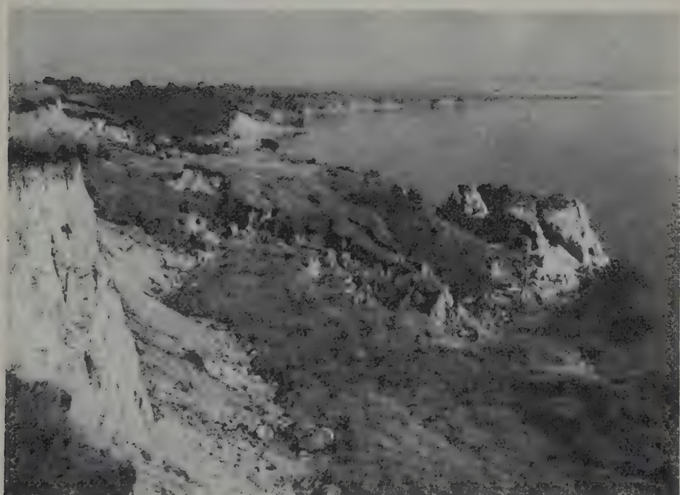
Fig. 1-16. Banks of the Nechranice reservoir in NW Bohemia affected by sliding (photograph by Záruba).
