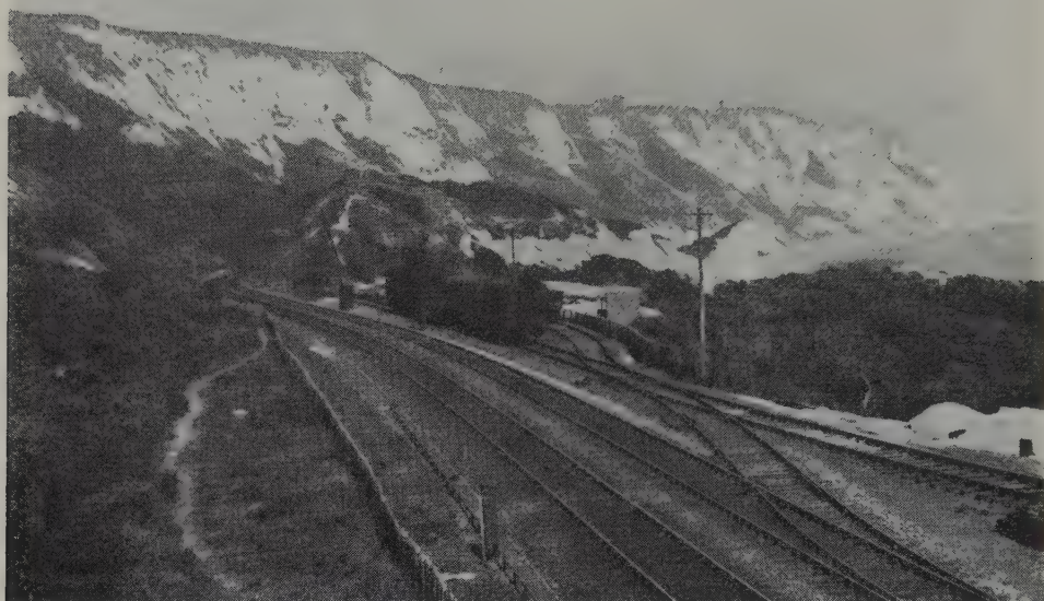
Fig. 5-31. Railway line near Folkestone threatened by sliding (photograph by Záruba).
