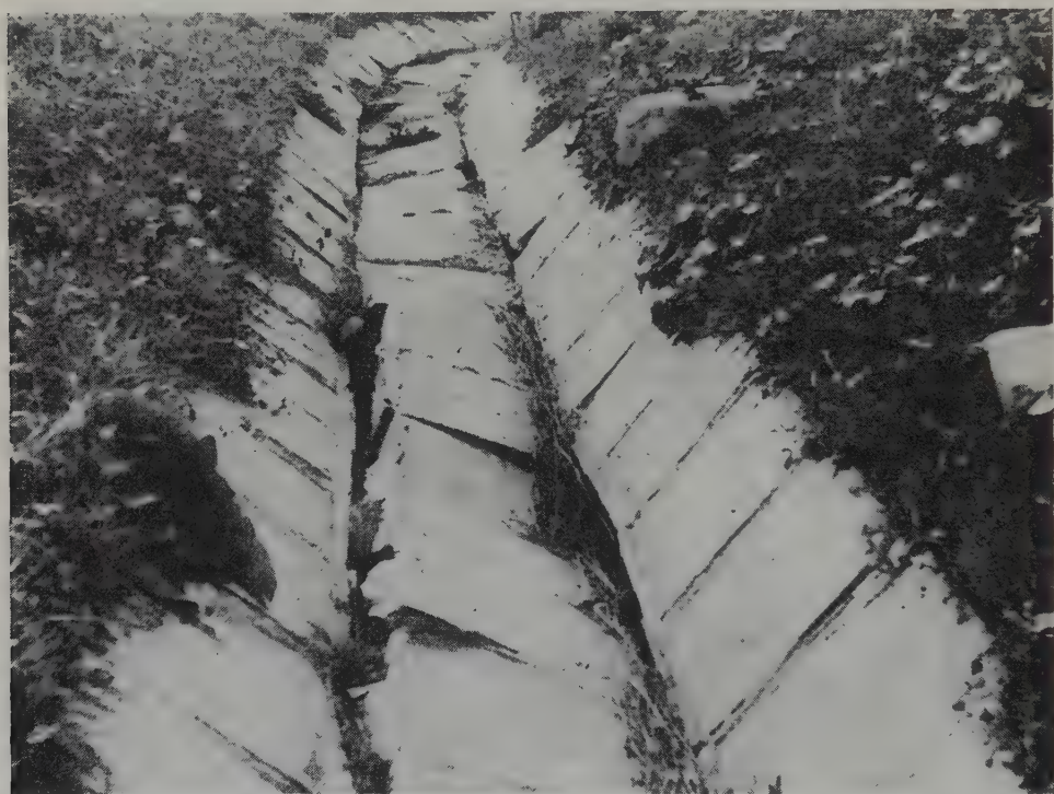
Fig. 8-8. Handlová landslide; continuous maintenance of the paving is necessary, as even small movements disturb the ditch and impair its function (photograph by Záruba).
