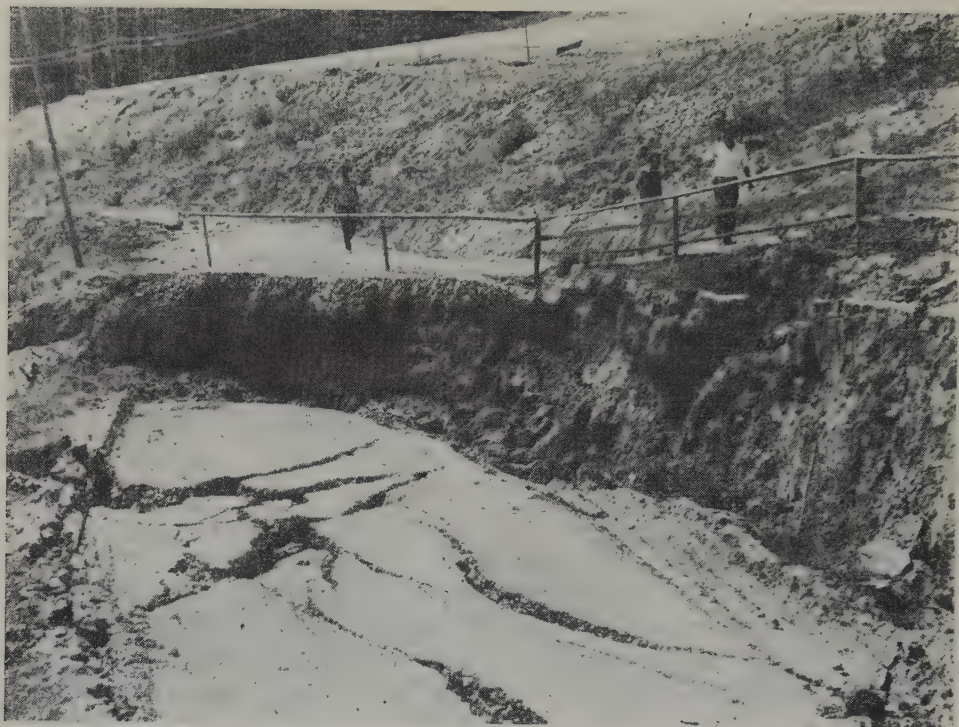
Fig. 1-10. Highway interrupted by landslide caused by excavation for dam abutment (photograph by Záruba).
