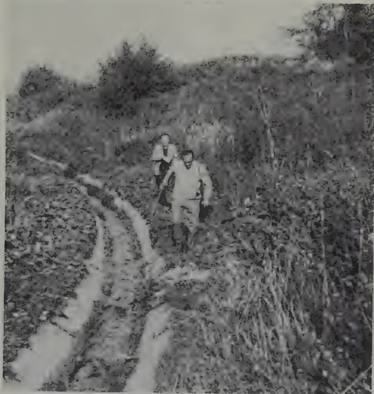
Fig. 8-7. Handlová landslide; drainage ditches paved with concrete tiles (photograph by Záruba).
