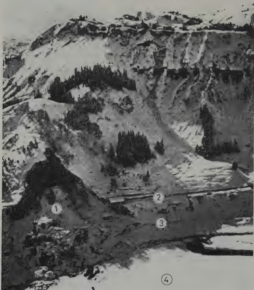
Fig. 1-13. The slope failure which destroyed the Takabayama tunnel in Japan, 1970; 1 — landslide in Neogene mudstone, 2 — railway line, 3 — highway, 4 — Shinano river (Japan Society of Landslides 1972).
