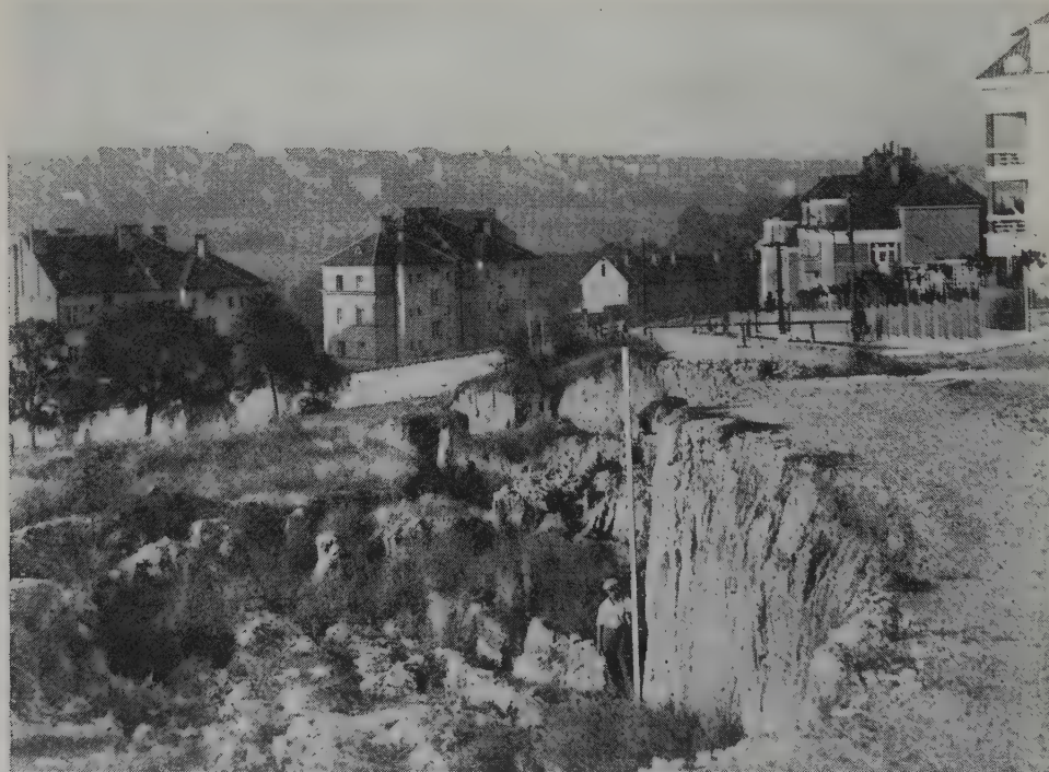
Fig. 12–11. Collapse of a steep slope of an abandoned loam pit in a suburb of Prague. Streets and buildings in the neighbourhood were damaged (photograph by Záruba).
