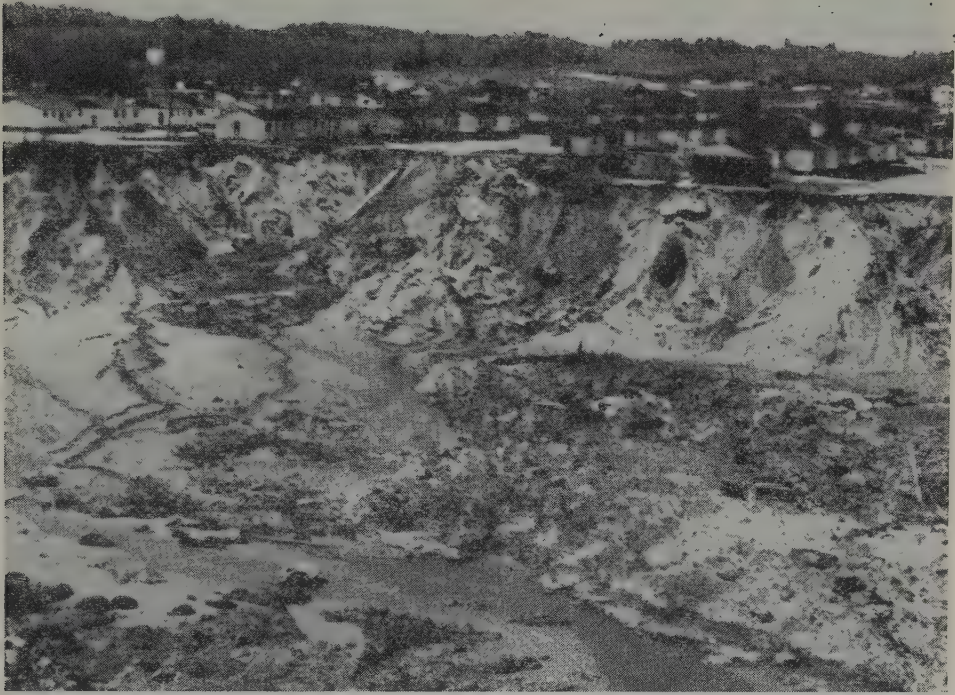
Fig. 1-4. Landslide in Leda clays at St. Jean Vianney near Quebec (Canada) in 1971. Forty houses were demolished and 31 people killed. (Courtesy Canadian Research Council).
